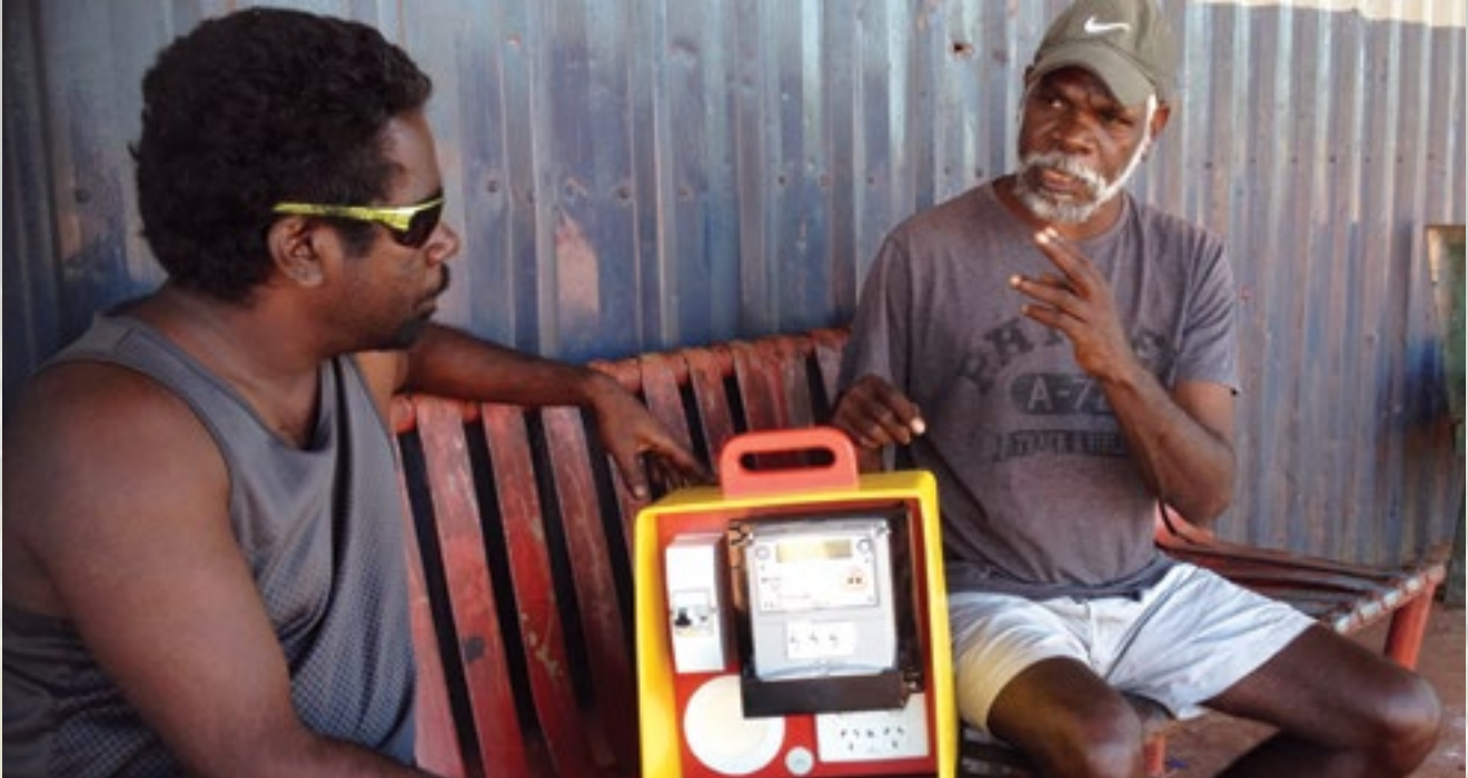
Above: Daniel Wunungmurra explaining the new meterbox to Timothy Dhurrkay Gurunja in Galiwin'ku.
